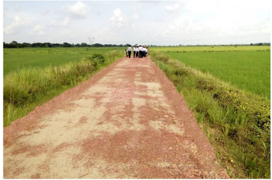
Construction of farm road in Kangyi village of Hlegue Township
