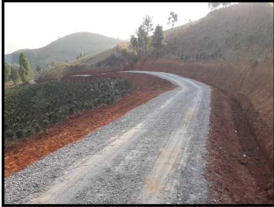
Construction of farm road in Ohm Ton Pin of Pintaya Township
