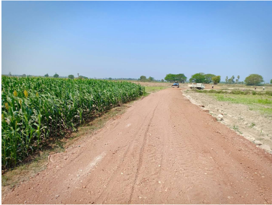
Construction of farm road in Yezagy Township
