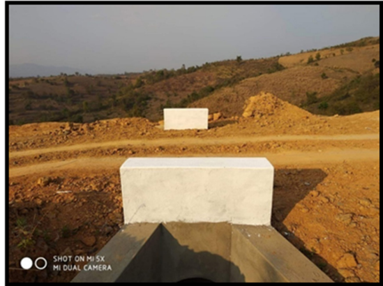
Construction of farm road and its pipe culvert in Mann Narr village of Lashio Township
